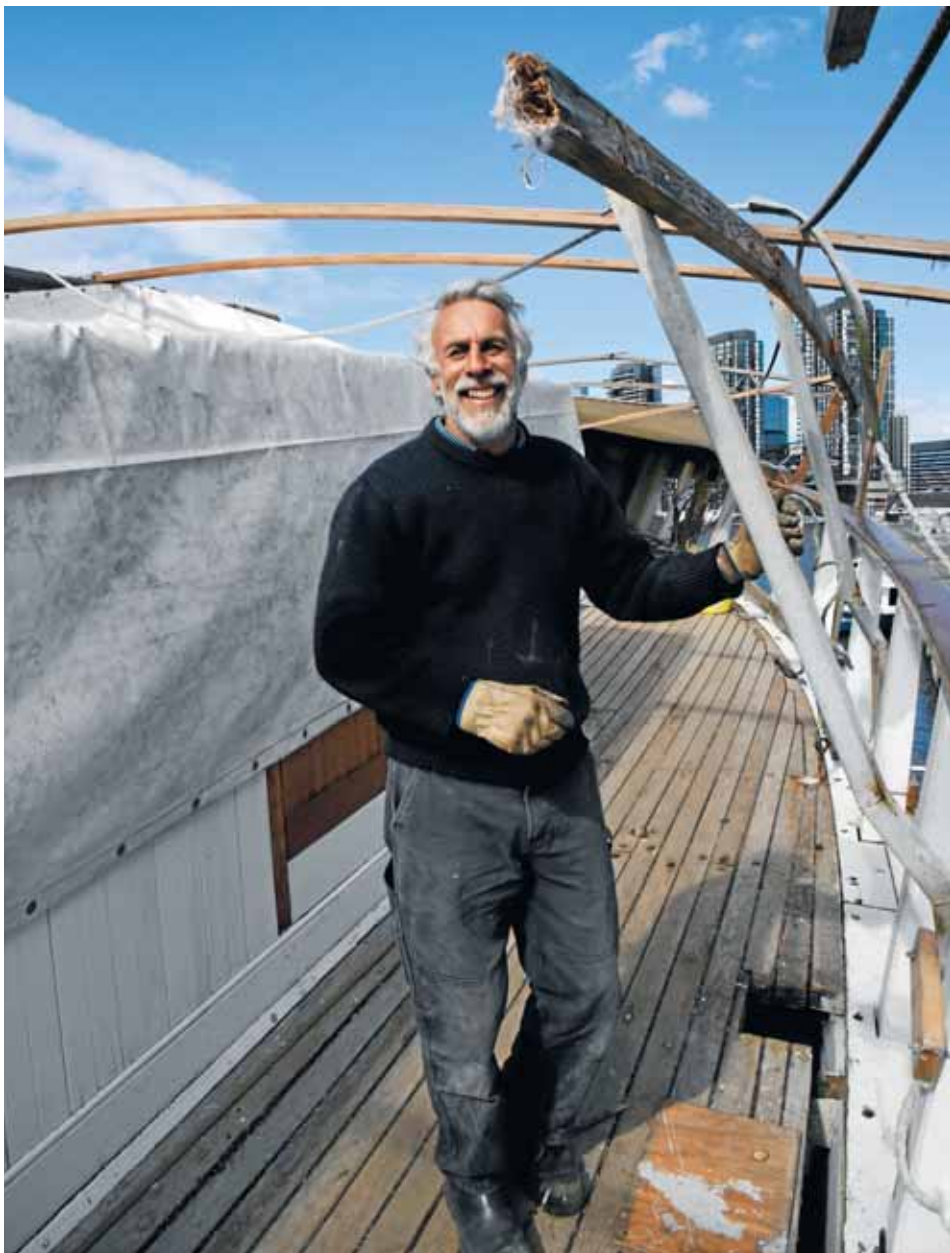
Project director Peter Harris gets on with repairing the storm damage.
