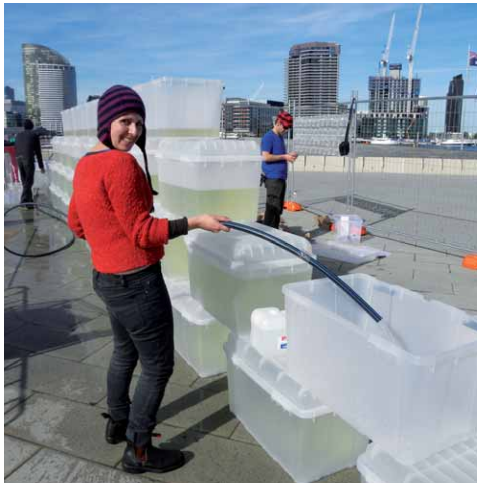
DirtyBuoys under construction half way through the 72 hours.
