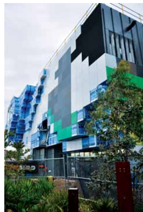
Works are almost complete on the new NBN Co HQ.
