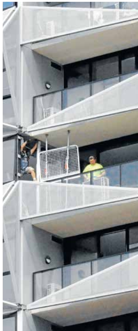
Workers removed non-compliant cladding from the Lacrosse building in Docklands.
