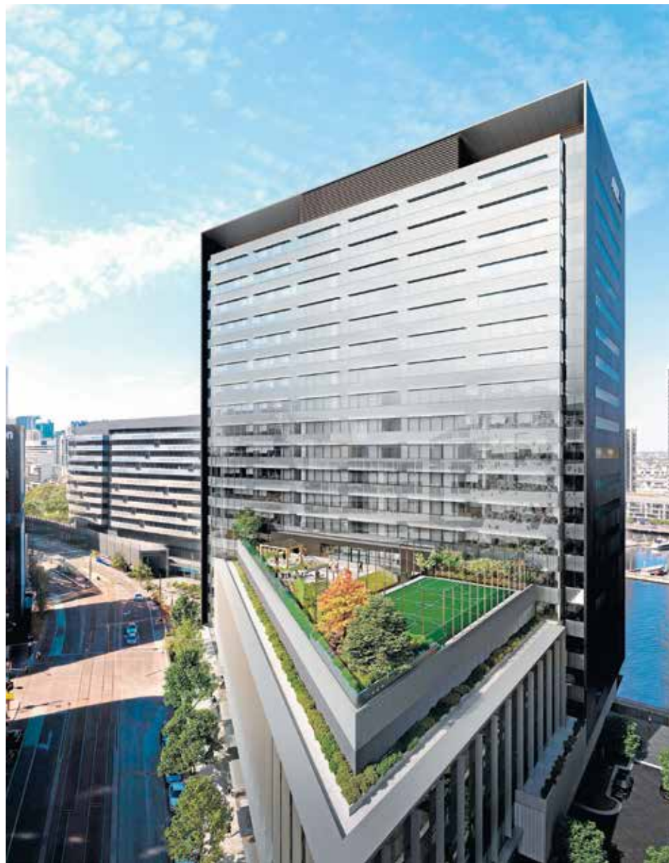
839 Collins St is on track for completion early next year.
