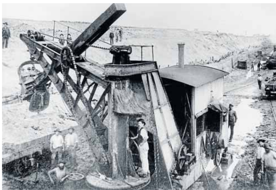
Work starts on the Yarra River diversion and Victoria Harbour excavation.
