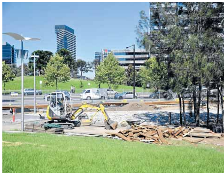
Upgrade work continues at the Collins St end of Docklands Park.
