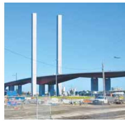
Construction of Ron Barassi Snr Park is nearing completion.
